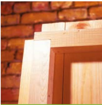
**1 The frame.** Decide how big you want your shed and plan dimensions accordingly. Construct four equally sized frames with half lap joints as shown. Cover the two side frames with tongue and groove boarding, using panel pins and glue. Leave a 60mm overhang on one side of each panel so that the next panel fits in flush.
