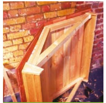
**4 The roof.** Glue & screw all frames together; the panels with triangular framed tops being the front and back of the shed. Clad the roof with tongue and groove boarding, then add roofing felt, or glue shingles to the boarding, overhanging all round, starting from the bottom up. (I've added a decorative timber support on the sides as shown). Arrange your tools in an orderly fashion!
