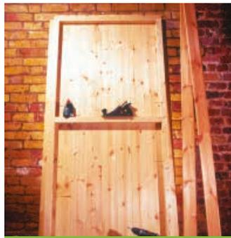
**2 The panels.** Trim the boarding off at the top of these two side panels. Make two triangular roof frames, with 30 degree angles, the bottom edge the same width as the shed. Glue & screw them to the top of the other two front and back frames and fit tongue and groove boarding as before, trimming the top edge to shape. Make sure all the panels fit together flush.
