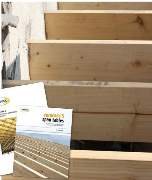
The load a member can carry depends on several factors, including its span, thickness, width and species. Usually, the deeper and wider the section, the longer the span.
