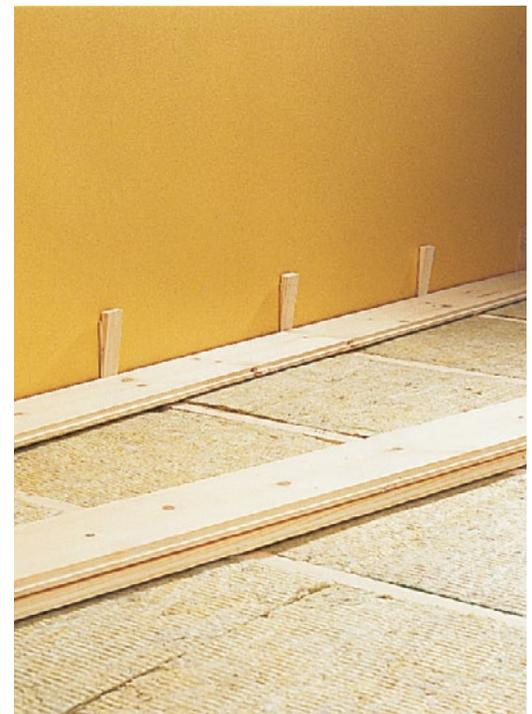
Leave an 8mm gap round solid wood floors to allow for natural movement. Cover with skirting boards.
